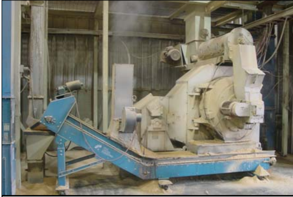
Wood peletizing mill in Arkansas
